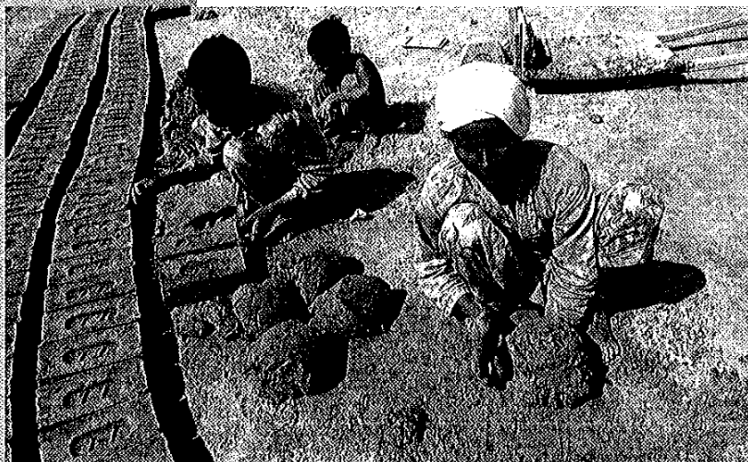
Figure 14-21 Young girls and boys work under scorching sun to construct this road in Batapur village, Pakistan.
